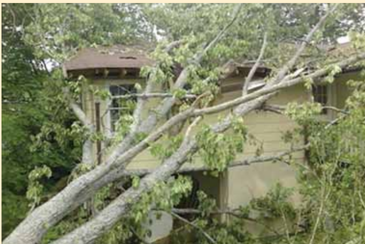
Damage to the home of Charline and Terry West in Tennessee.
