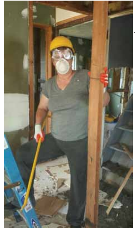
Carol Liesch, I.I.I., was part of the demolition crew.
